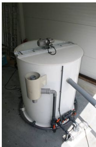
To the left flotation chamber in PE, above Adoxpol Ozone system
