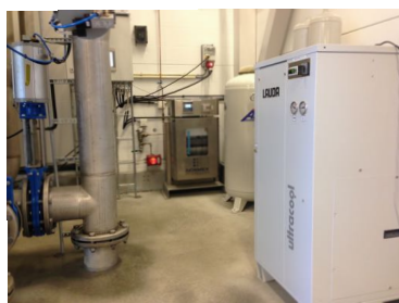
To the left flotation chamber in PE, above Adoxpol Ozone system
